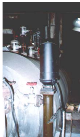
Level Controller c/w chamber
